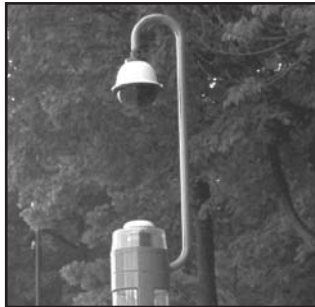
The weather resistant QFD is being used at all Illinois interstate highway rest areas, part of the state's Homeland Security initiative.
